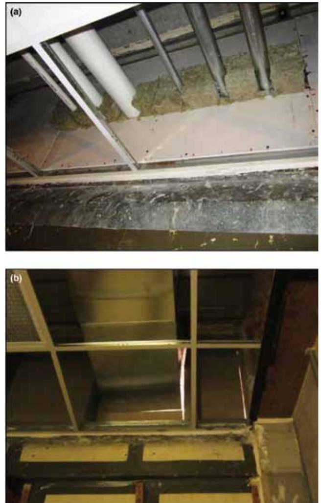
Figure 4. A quick installation technique was used for some of the drywall barriers: (a) large openings were left around the penetrating elements so simple rectangular pieces of drywall could be used; those openings were stuffed with pieces of stone wool insulation; (b) large gaps between pieces of drywall and around the penetrating elements were not caulked or taped; light shining through the gaps from the opposite side of the barrier show their size and extent.
