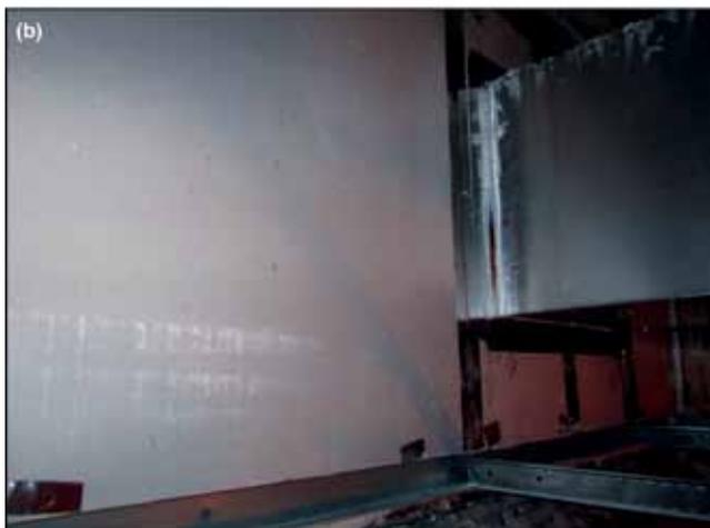
Figure 5. A sealed installation technique was used for some of the drywall barriers: (a) drywall was cut closely around the penetrating elements and caulked; (b) joints, screw heads and penetrations were sealed with metal tape.
